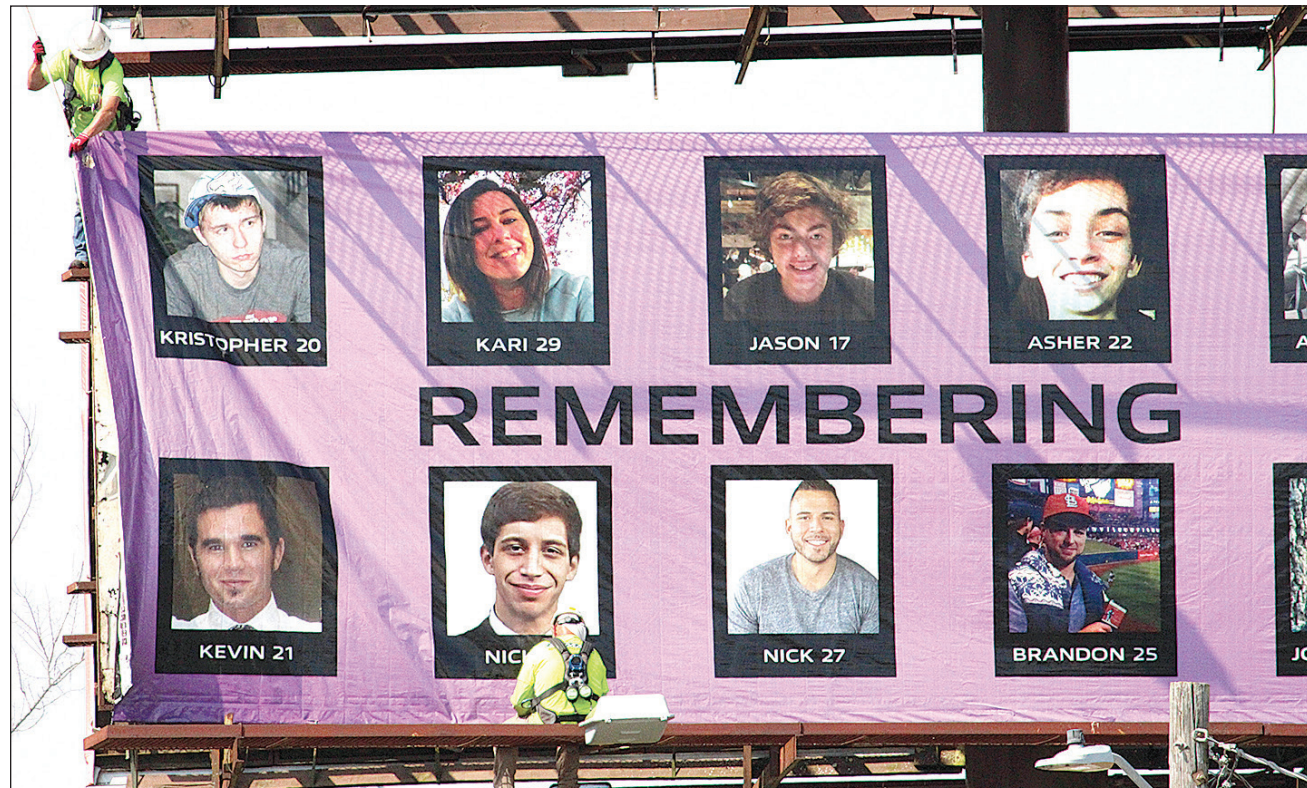
Workers finish setting up one of the new billboards along Interstate 70 in Warrenton. This one contains the picture of Kristopher, the nephew of Sabrina Wipfler who is using the billboards to raise awareness about the heroin epidemic.
