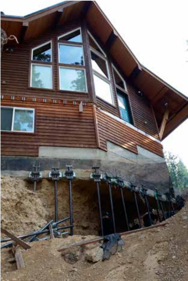
Foundation stablization associated with a residential landslide mitigation project, Chelan County.
