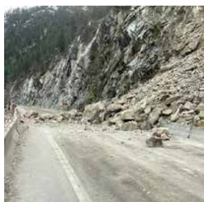
COURTESY OF WSDOT A slide at milepost 10.7 overflowed the catchment basins and crossed both lanes of the road on Monday, March 3.
