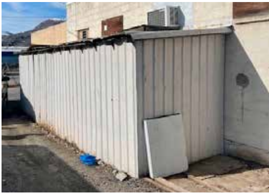
MIKE MALTAIS/WARD MEDIA The metal roof on the storage space attached to the south side of the Center building needs attention to stop water leaks.
