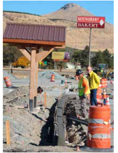
MIKE MALTAIS/WARD MEDIA A fresh concrete footing cures behind the information kiosk installed by the Okanogan County Tourism Council earlier this year.
