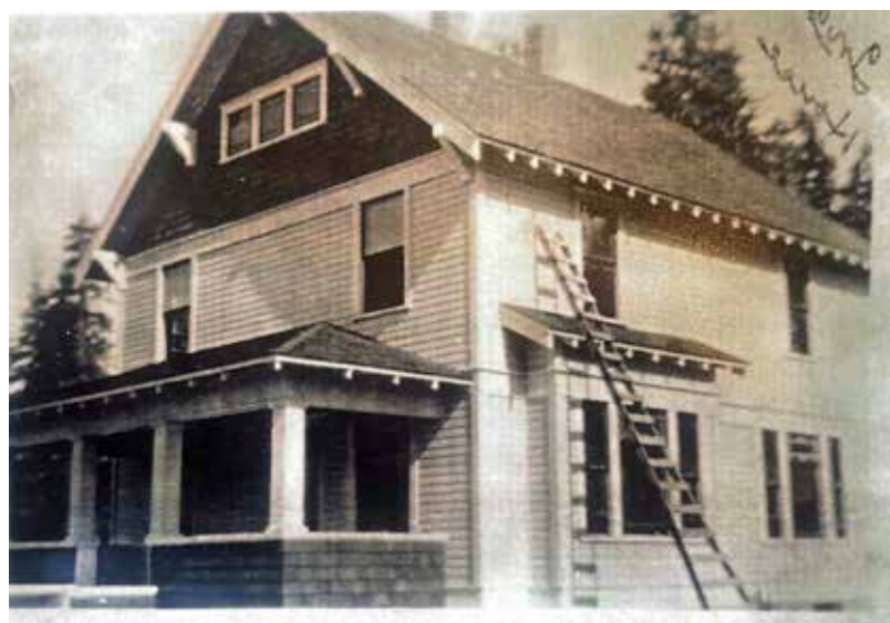
COURTESY OF BILL BURGESS The house in its early years. The scanned photograph has been flipped to accurately reflect the position of the house.
