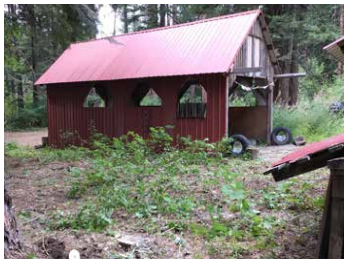
Properties after receiving fuels reduction work.
