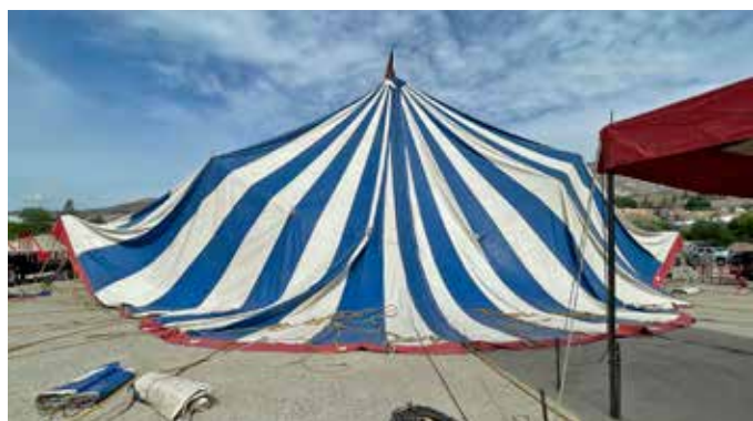
The 30-foot center pole is set.
