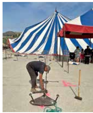
Support cables stabilize the structure.
