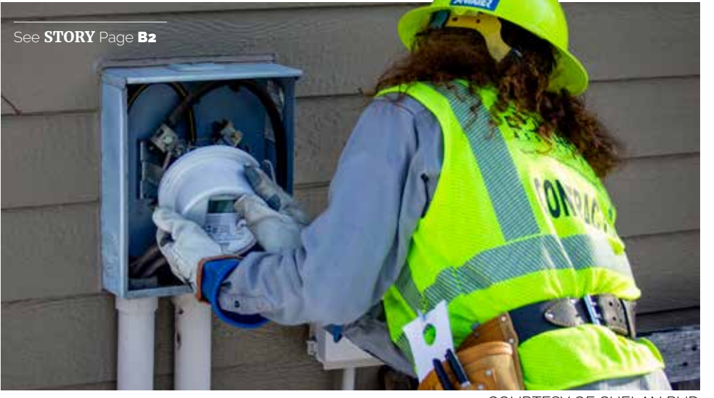
Chelan County Public Utility District is in the final stages of replacing traditional electric meters with advanced metering infrastructure throughout the county.
