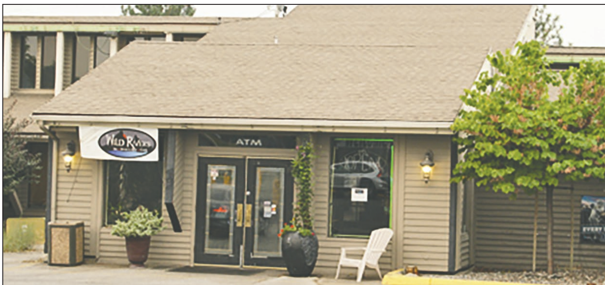
The Wild River Inn was not renovated, but was included in the original purchase of the hotel last year.
