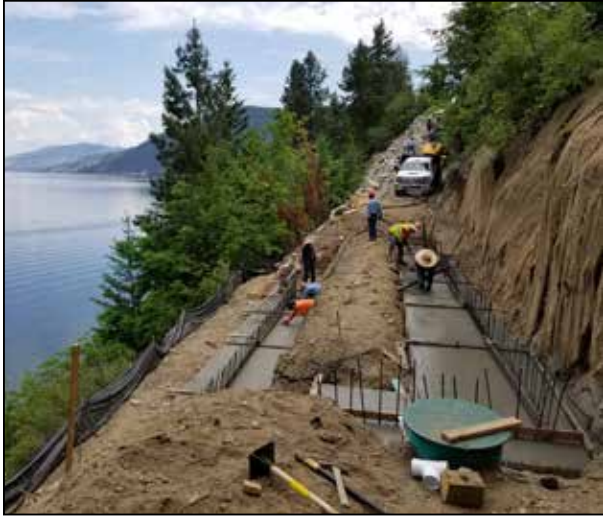
Legion Concrete works on the job.
