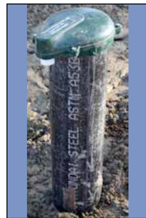
The end result is a wellhead ready to have a pump installed.
