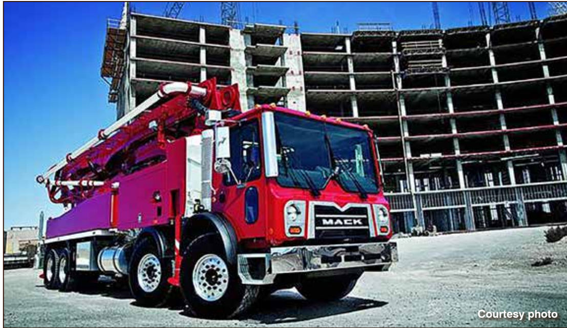
Cement truck at job site.
