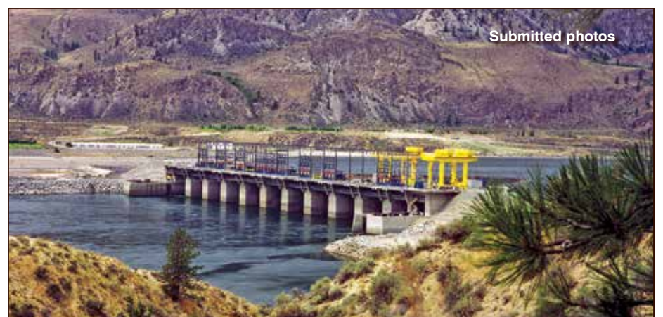
Wells Hydroelectric Project.
