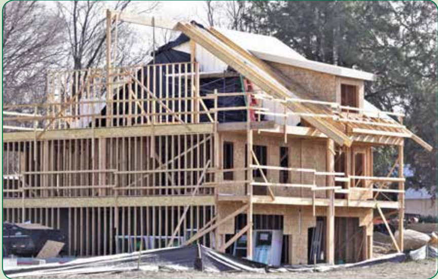
Construction has begun.
