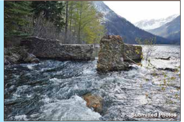
In the spring of 2018, floodwaters and runoff overtopped Eightmile Dam.
