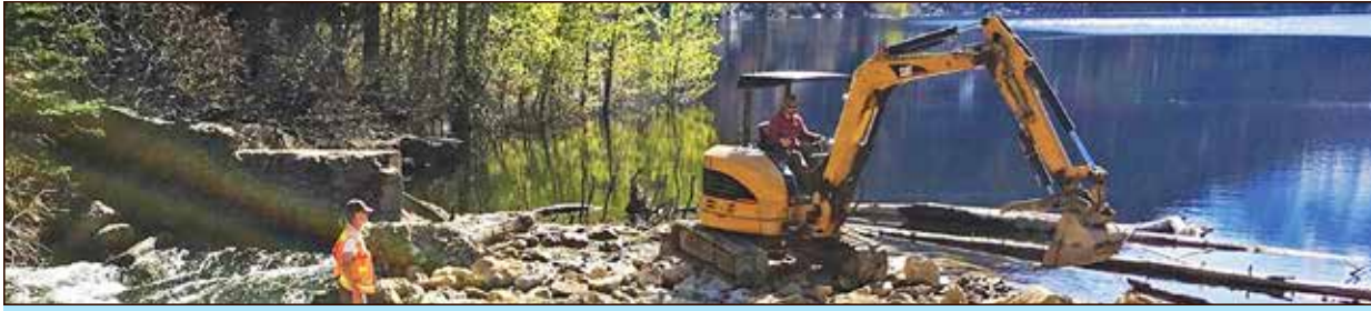
Emergency temporary construction at Eightmile Dam.
