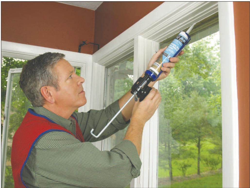
BPT Photo Caulk around windows and doors - Air can also leak through minute cracks around windows and doors.
