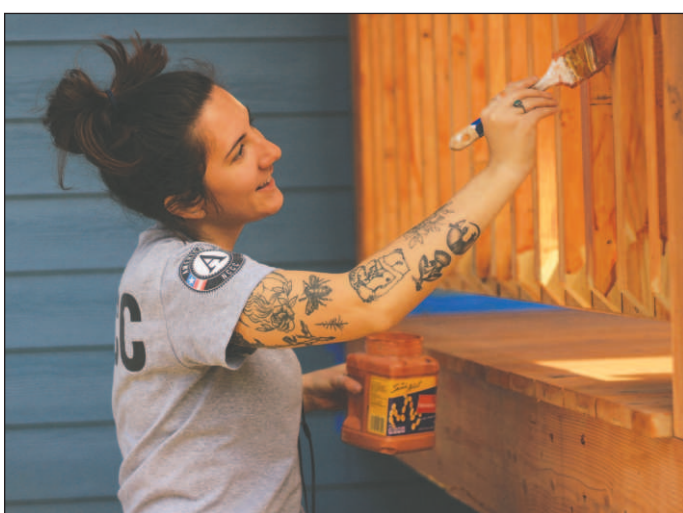
Anna Pleskow, one of the 11 AmeriCorps NCCC Green 3 team members working with the Okanogan County Long Term Recovery Group, applies stain to a deck rail.
