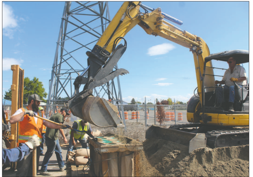
A Rains Contracting crew uses a gang frame of plastic pipe sections to fill 10 sand bags at a time with a front-end loader in Columbia Cove park. The bags are being used as part of a shoreline stabilization project along Columbia Cove Park.
