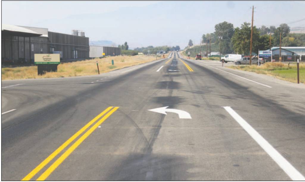
Photo by Mike Maltais Department of Transportation crews from Wenatchee completed the installation of a new two-way left turn lane along this stretch of U.S. 97 at the Brewster-Grange Road west of Brewster last week. The new alteration is designed to reduce the incident of accidents in the high traffic area.
