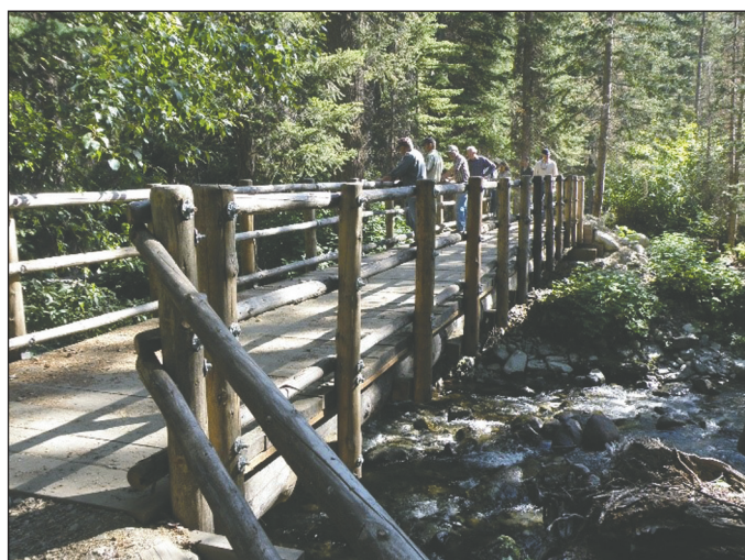
USDA Forest Service/ Robin DeMario Forest Service employees and Resource Advisory Committee members stand on the reconstructed South Creek Bridge located on the Methow Valley Ranger District. Backcountry Horsemen volunteers, working with Forest Service personnel, reconstructed the bridge using Secure Rural Schools Title II funds.
