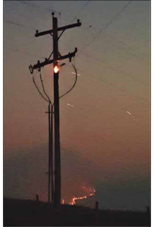
With flames visible on Dyer Hill in the background across the Columbia River, embers near the lower spar of a utility pole glow in the dark and release sparks in gusts of wind on the Colville Reservation.
