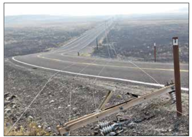
Downed utility wires stretched across a section of Road E N.E. southeast of Mansfield where flames damaged or destroyed many power poles.
