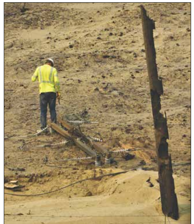
A utility worker inspects the top section of a power pole that burned along Road B N.E. between Bridgeport and Mansfield.
