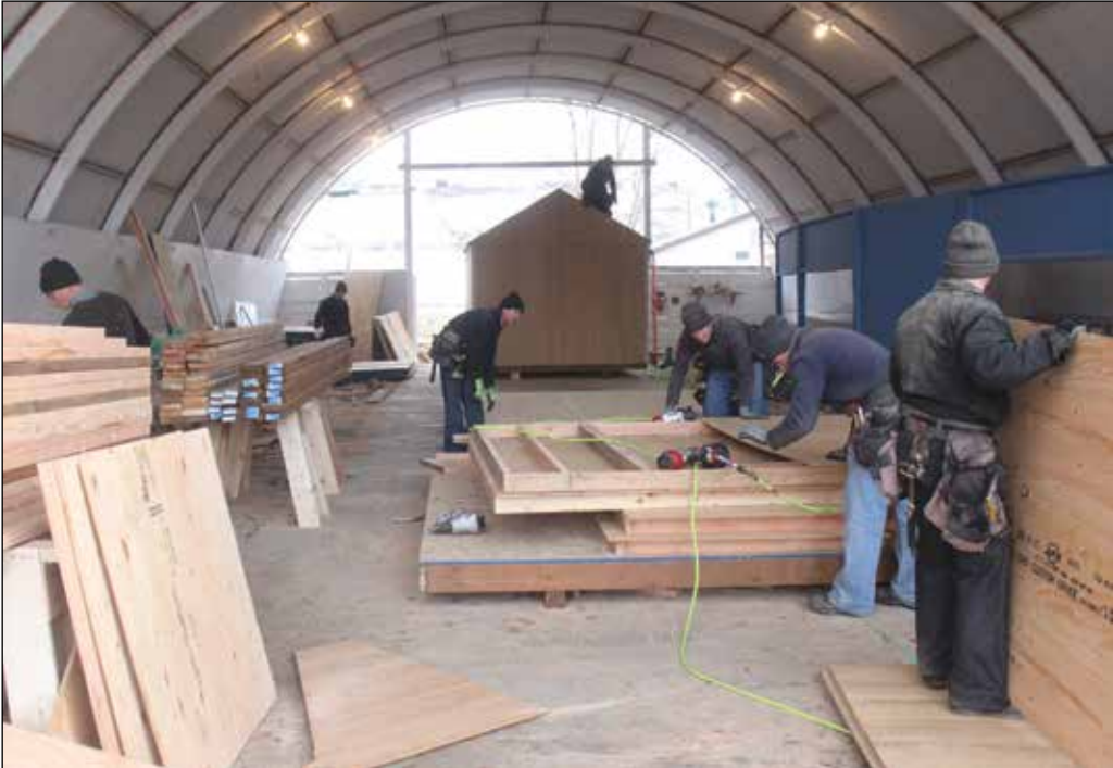
WAMS builders employed an efficient assembly line-like system to construct sheds in one of the livestock Quonset buildings on the Okanogan County Fairgrounds.
