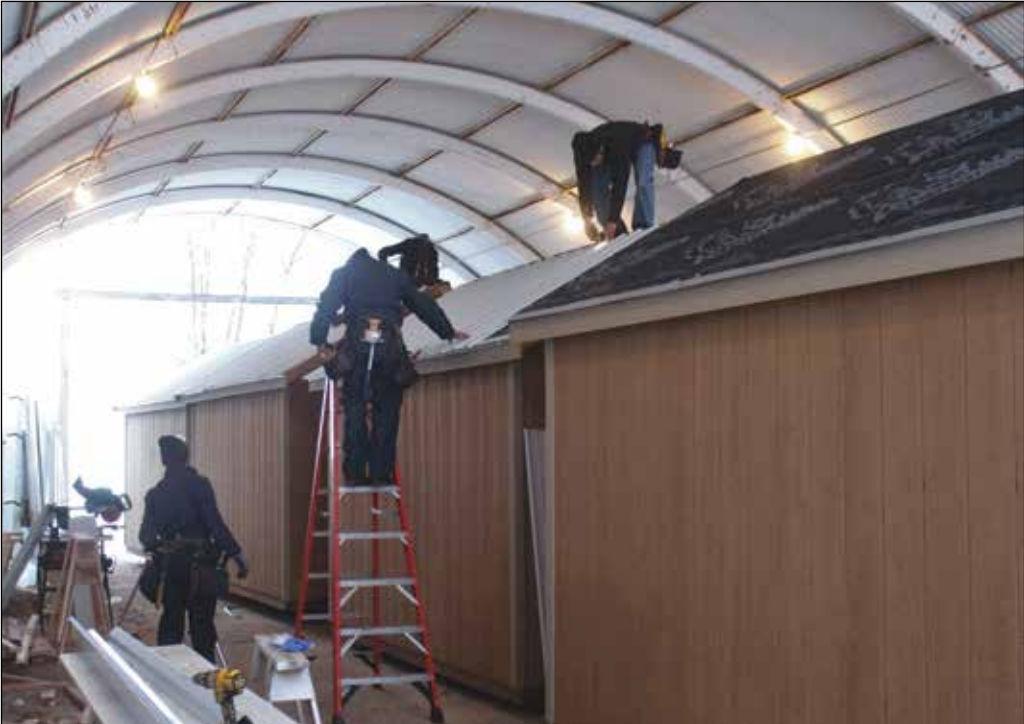
The finished sheds were returned by forklift from the outdoor staging area so volunteers could apply the final step of metal roofing to each unit. More photos at qcherald.com
