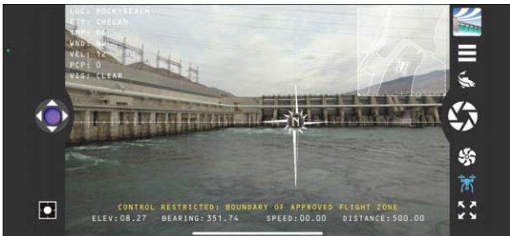
Using the new PowAR app, guests can use augmented reality to "fly" a drone over Rocky Reach Dam.
