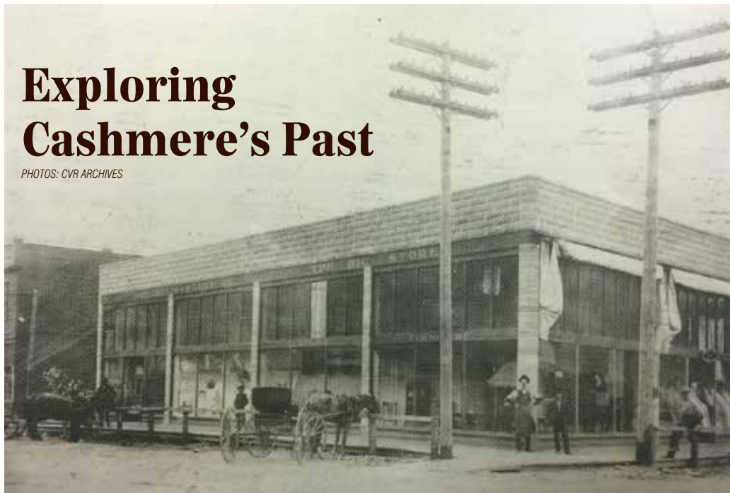
Ellis-Forde building in 1908
