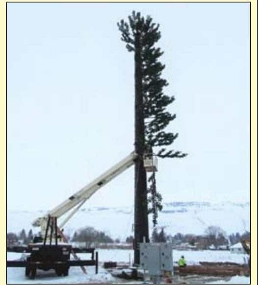
Courtesy Ken Krugel A new twist on the term "phone tree" practically sprouted overnight along Fairview Avenue in Bridgeport as AT&T workers erected this monopine 5G cell phone tower and added branches designed to disguise its intended purpose.
