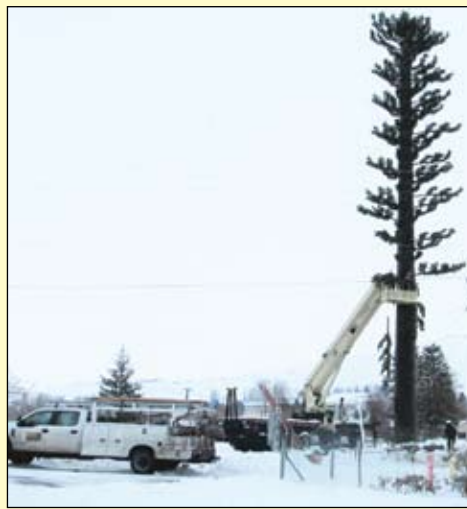
Courtesy Ken Krugel A new twist on the term "phone tree" practically sprouted overnight along Fairview Avenue in Bridgeport as AT&T workers erected this monopine 5G cell phone tower and added branches designed to disguise its intended purpose.
