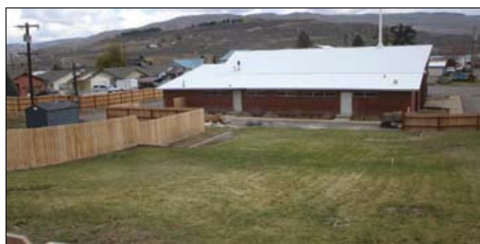
A previous AmeriCorps crew built this wood fence around the Treehouse property.
