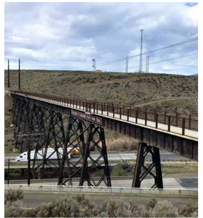
The Renslow Trestle over I-90
