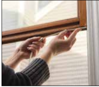
Courtesy StatePoint Fill the Seals. Reinforcing the seal around the entire window frame will ensure it's ready for cold weather.
