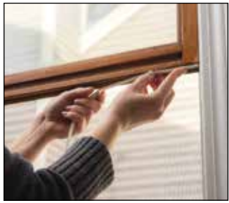
Courtesy StatePoint Fill the Seals. Reinforcing the seal around the entire window frame will ensure it's ready for cold weather.
