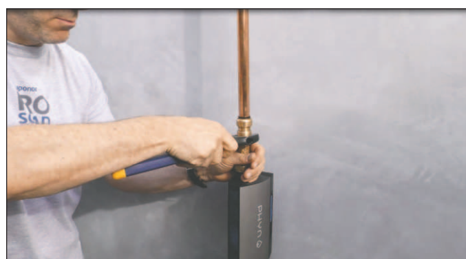
©BPT Installed right after the water meter, the Phyn Plus smart water assistant + shutoff automatically measures tiny changes in water pressure in the home's water supply lines, 240 times per second, to identify and alert homeowners the moment a leak is detected.
