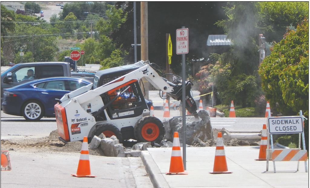
WSDOT workers digging the ground in front of Cashmere Valley Bank where one of the two bulb outs will be constructed.
