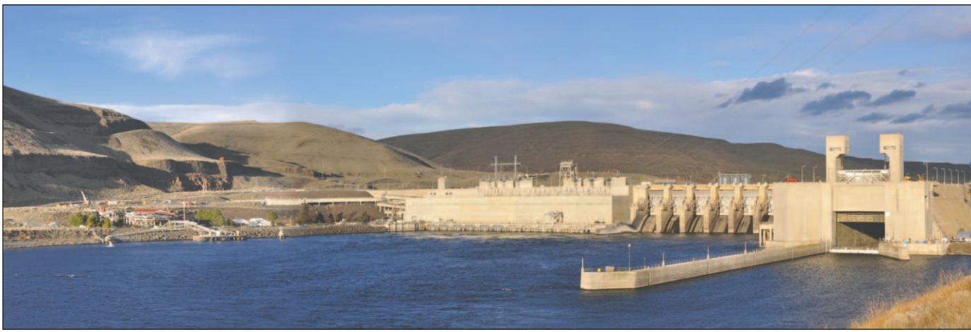
Lower Monumental Dam on the Snake River.
