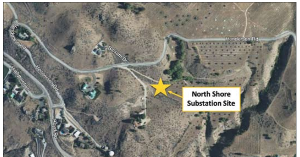
Construction on a new substation to serve growth and development on the north shore of Lake Chelan will begin this month on Henderson Road.
