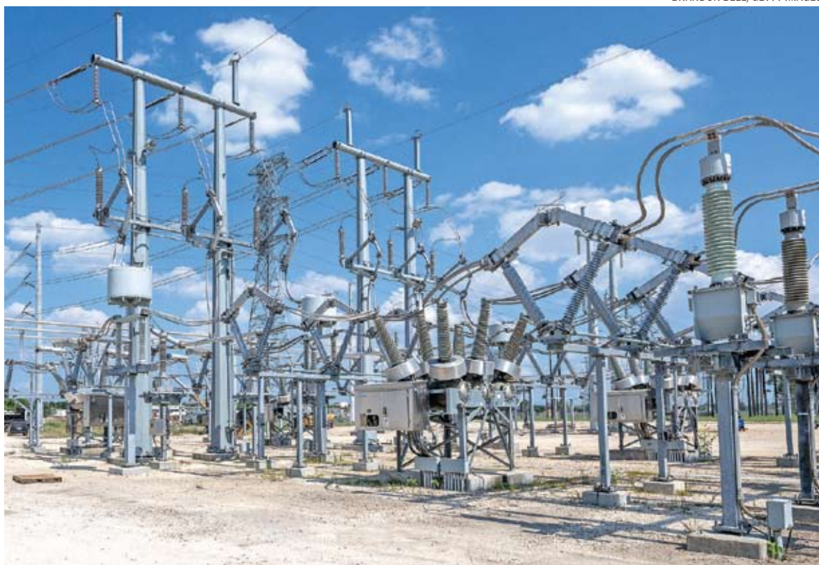
▲ An electric generator in Houston on June 9, 2022.
