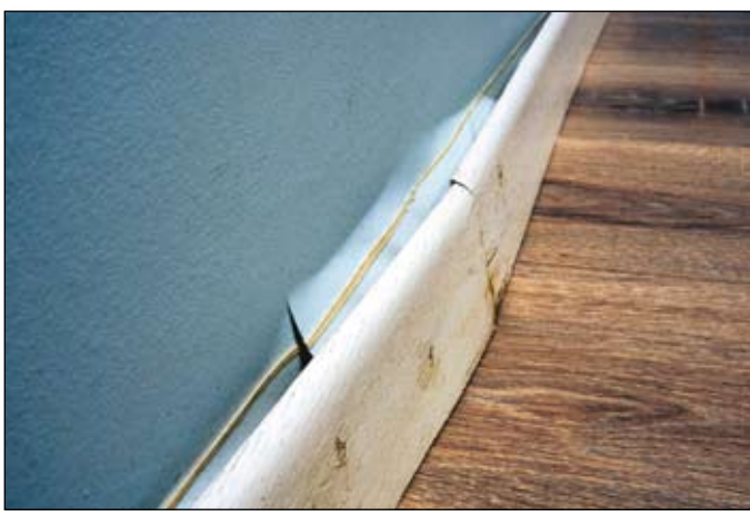
PHOTO SOURCE: (c) designer491 / iStock via Getty Images Plus FEMA says floodwater only needs to get a mere 3 inches high to make it likely that you'd need to replace drywall and baseboards.
