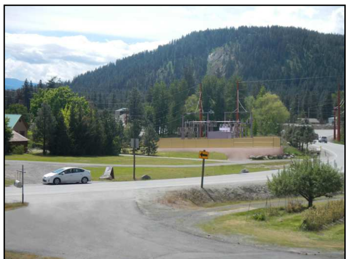
Photo submitted by Teka Sellers The Chumstick location seems to provide that best cover to hide the substation from public view.
