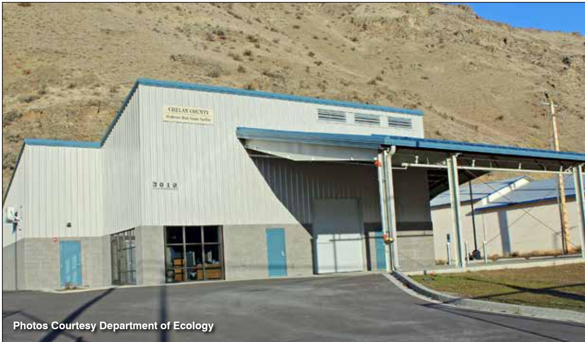
The new Moderate Risk Waste Facility.
