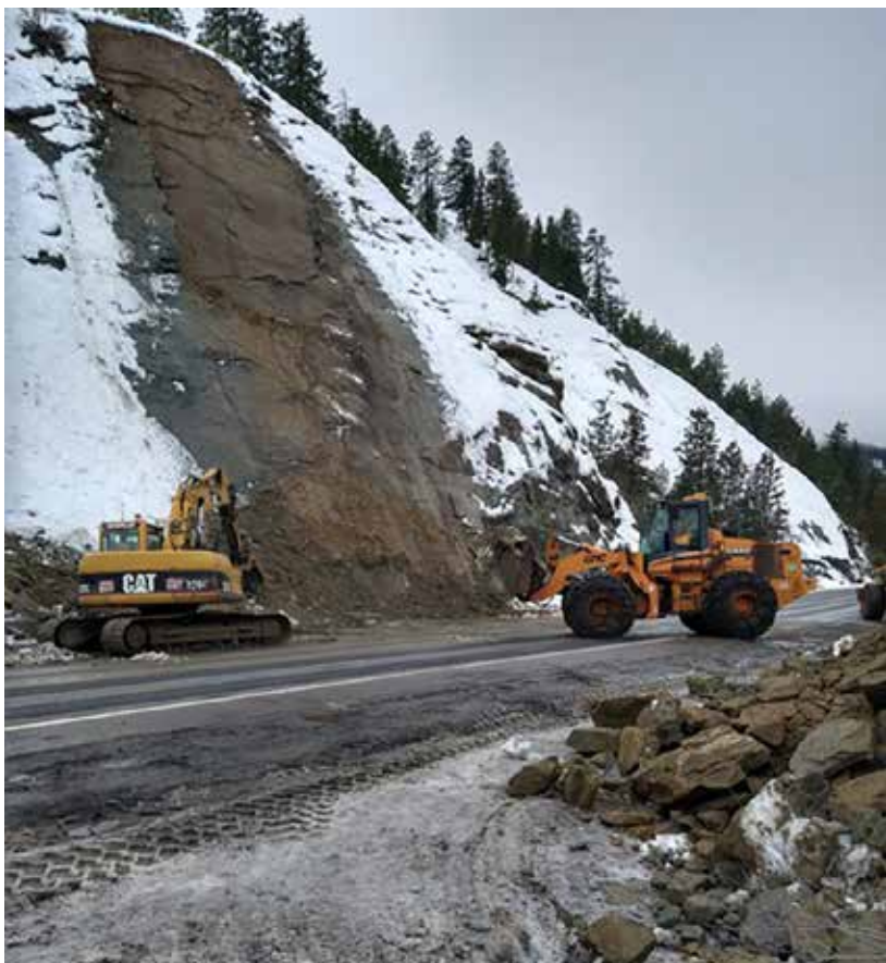
PHOTOS COURTESY OF WSDOT.
