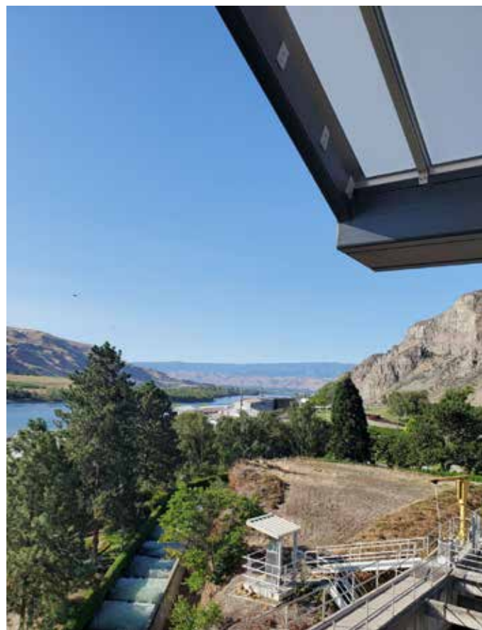
Improved view of the fish ladder and Columbia River from the new observation deck
