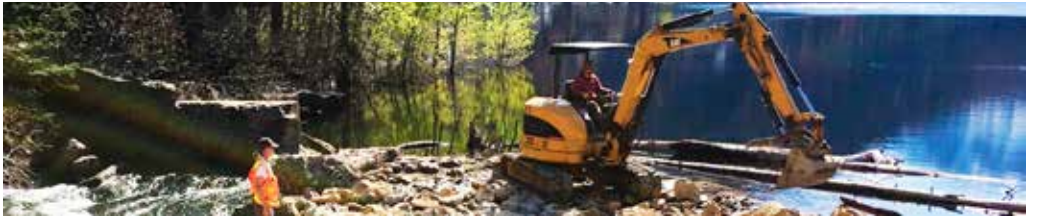
Emergency temporary construction at Eightmile Dam
