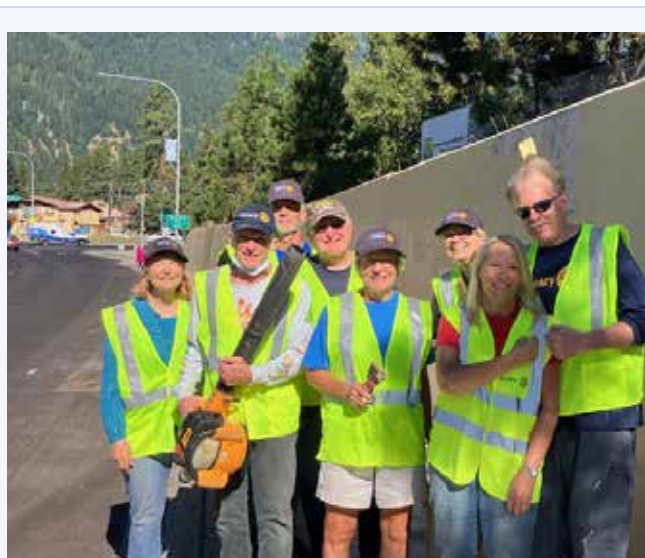
Leavenworth Rotarians are getting ready to paint the wall on Hwy. 2. The paint and equipment were donated by the City.
