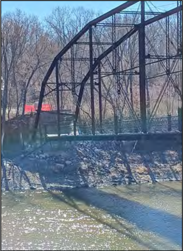
On Feb. 27th, the bridge over the Skunk River in northwest Lee County has slipped off its southern abutment and is sitting on the embankment about 12 feet below where it was previously.
