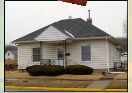
3BR • 1BA • 1 car garage 928 sq. ft. • 1,087 sq. ft. lot Very nice maintenancefree home by Lincoln School with a 75 X 145 fenced yard, nice patio, fire pit and child's play set! Some very nice built-ins, some original hardwood flooring, full basement including laundry area. Also find extra parking, garage and carport area on the paved alley. Listing #20164148 • $72,500
