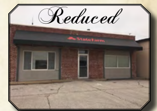
939 Avenue G Turn Key Office Space Listing #20165675
