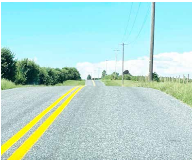
An example of a finished chipseal pavement in rural Pennsylvania. COURTESY PHOTO
