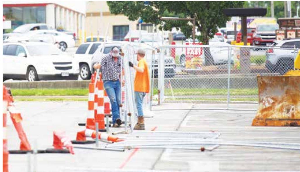
Kansas Fencing Inc. employees set up barricades around the southwest corner of Walmart Supercenter parking lot as construction commenced this week for Panda Express. Commissioners initially approved the short-form plat submitted by RTM Engineering Consultants for the restaurant, to be located at 27th St. and Broadway, at a Pittsburg City Commission meeting on Sept. 14. AARON PYLE / THE MORNING SUN
