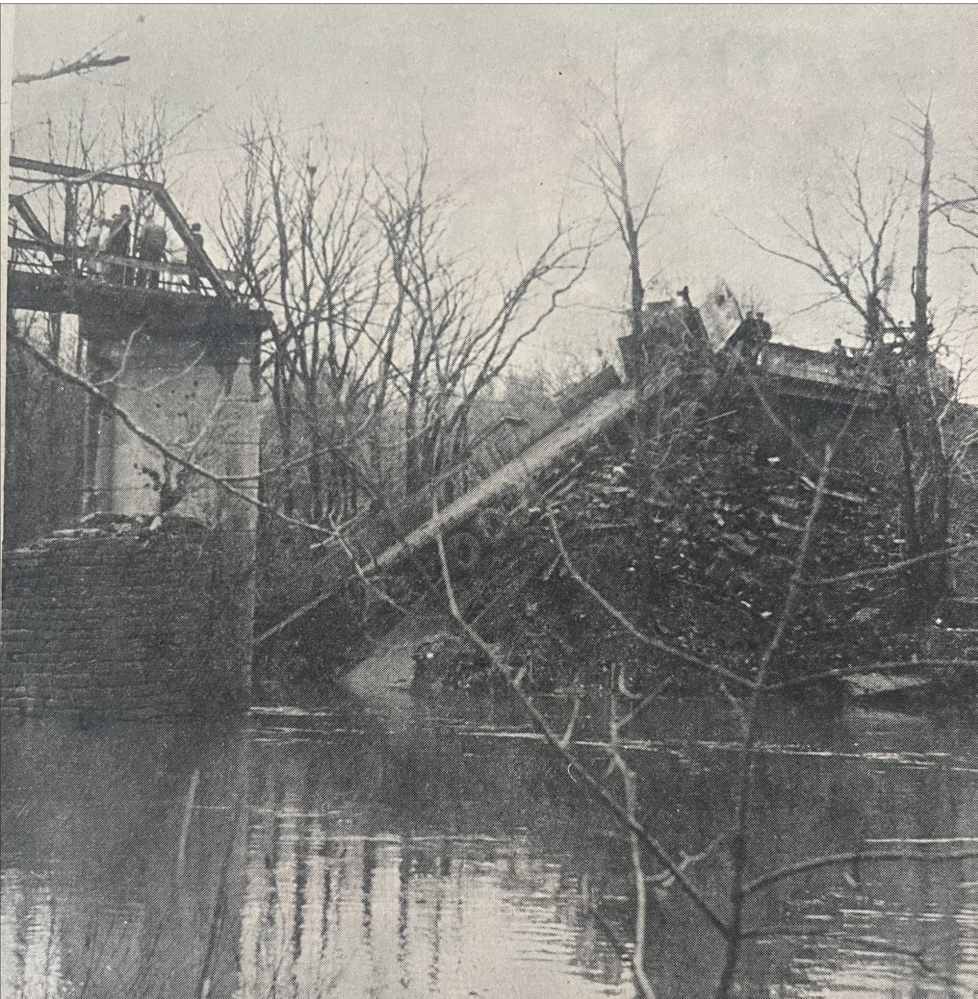
Duck River bridge between Verona and Caney Spring collapsed as a truck carrying 42 tons of cargo attempted to cross. (from The Marshall Gazette, Feb. 10, 1970.)
