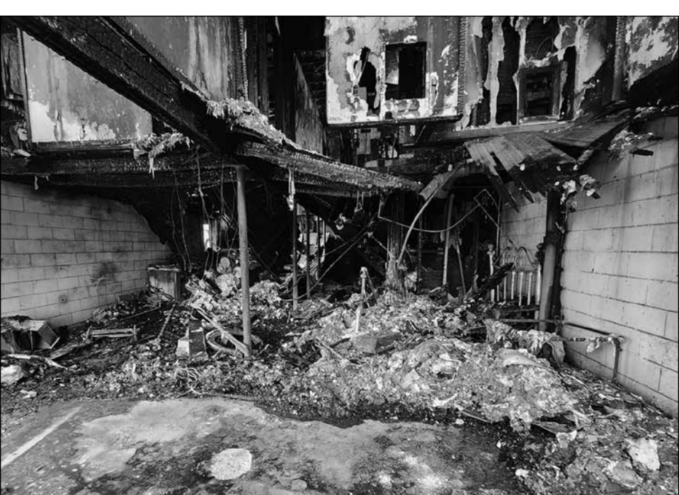
Ashes are left in the garage of the Apple Street home.
