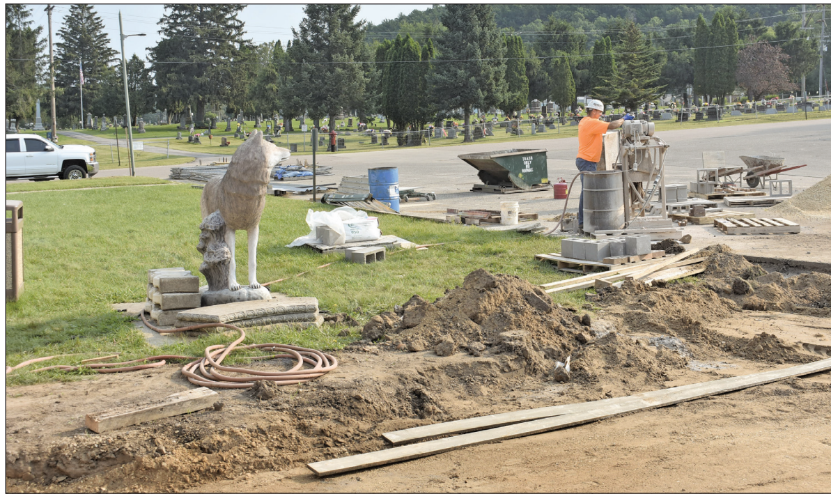
Contractors have been working outside Wonevoc-Center Schools to install a new concrete patio area, where students will be able to spend their lunch hour outside if they desire. Photo taken by Nicolette Nauman, HSE Editor.
